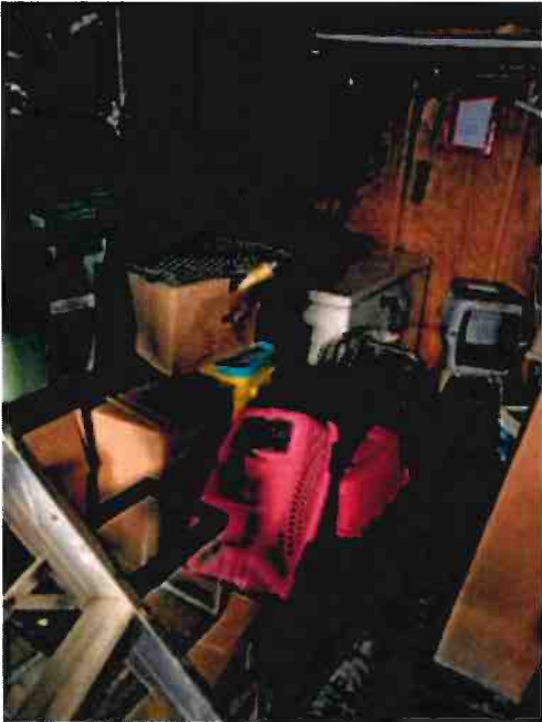
The freezer to store animals that have been euthanized is way in the back of a storage shed and the wood floor is deteriorating
