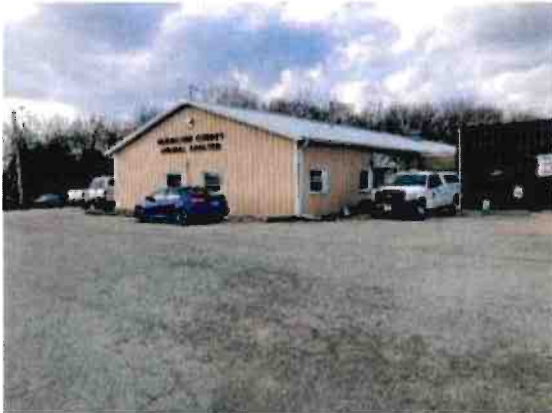
Front view of existing shelter
