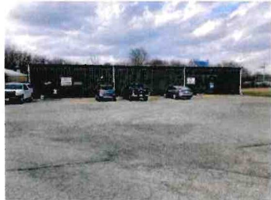
Front view of existing shelter
